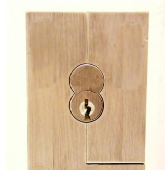
Interchangeable Core Cylinder
