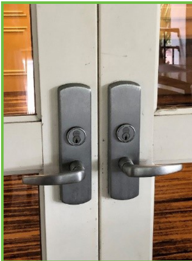
Hardware unlatched by a rotational motion is required by the 2021 I-Codes to operate with a maximum of 28 inch-pounds of force.
